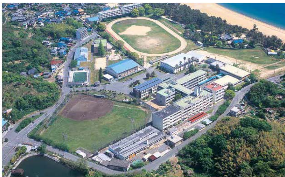
校舎地区全景 [Areal View of the School]
